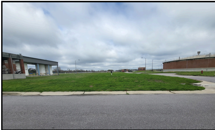
Future site for the Dewatering Roll Off Receiving Station structure.
