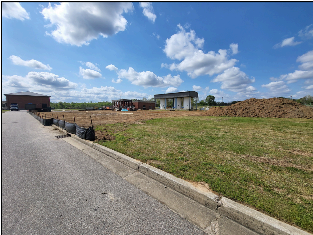
Site work underway with stockpiling of soils and erosion protection.
