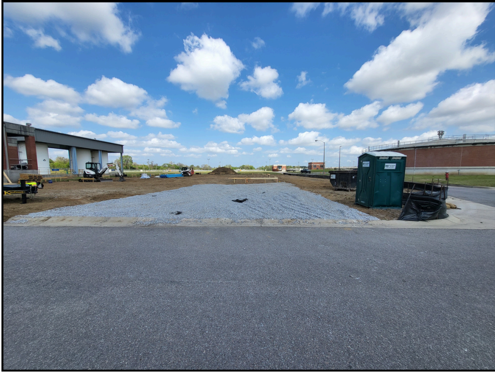
Construction entrance installed and equipment provided as the work begins.
